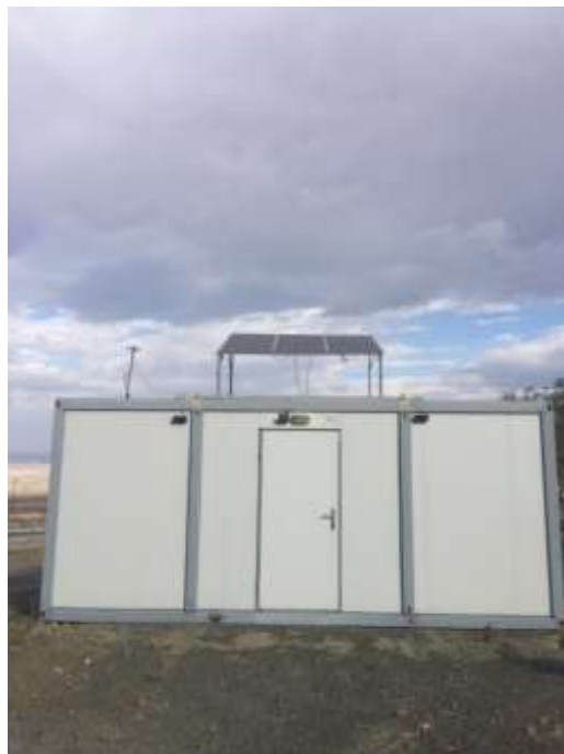
Figure_14: PV Photovoltaic Solar Panel Modules.
