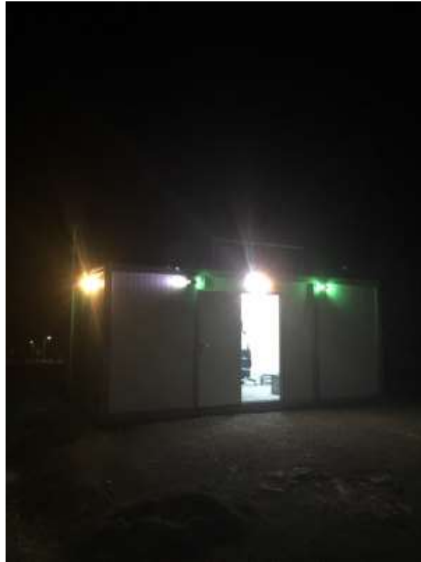
Figure_19: The solar PV panel module and wind turbine produce lighting electricity at the night time.
