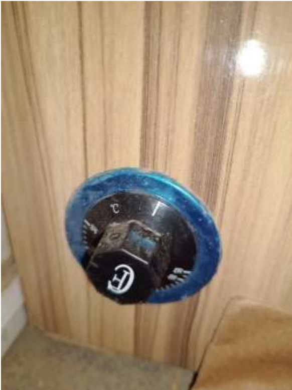
Fig. 3. The switch that is responsible for increasing the temperature of the whole system also serves as the switch for powering the whole system if the switch is on from the control box
