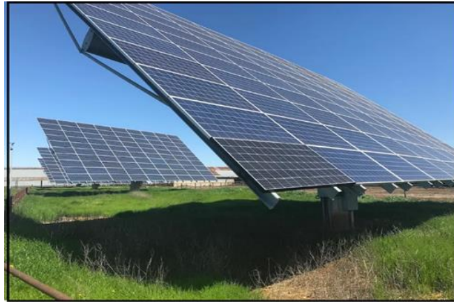
Fig. 7: dual-axis solar tracker
